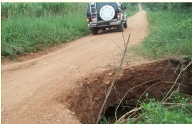
**Figure 3:** A damaged Kalagala- Kiziri road soon after construction (Credit: ACODE Digital Library)
