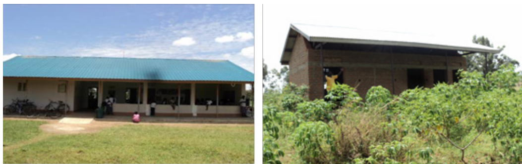
Figure 3: Poyameri HCIII in Magoola built by World Vision and Apuwai HC II, which has been in this state of disrepair for four years due to the contractors' failure to complete the job
