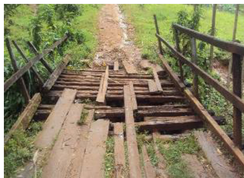
Figure 6: A dilapidated Nakatsi-Nabweya Bridge and Nalwanza – Bumusi Road
