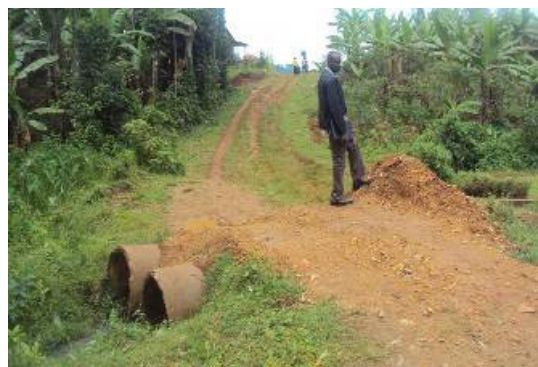
Figure 6: A dilapidated Nakatsi-Nabweya Bridge and Nalwanza – Bumusi Road
