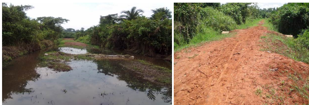
Figure 7: Left: An impassable community road (Kikugi) in Kakiri Sub-county (during the previous assessment). Figure 8: Right: The current state of Kikugi road (during the FY2012/13 assessment)
