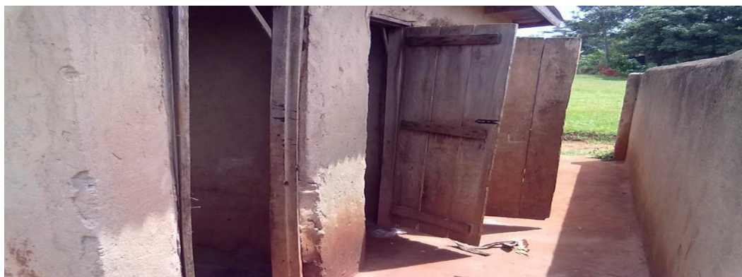
Figure 5: Dilapidated boys' latrine stances at Kabbabi-Bulondo Primary School, Mende Sub-county
