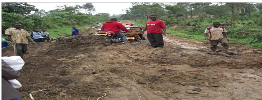
Figure 9: One of the roads in Namayumba Sub-county in a poor state
