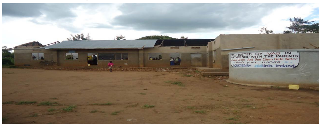
Figure 4: Part of the roof that was blown off at Naguru Primary School, Masuliita Sub-county
