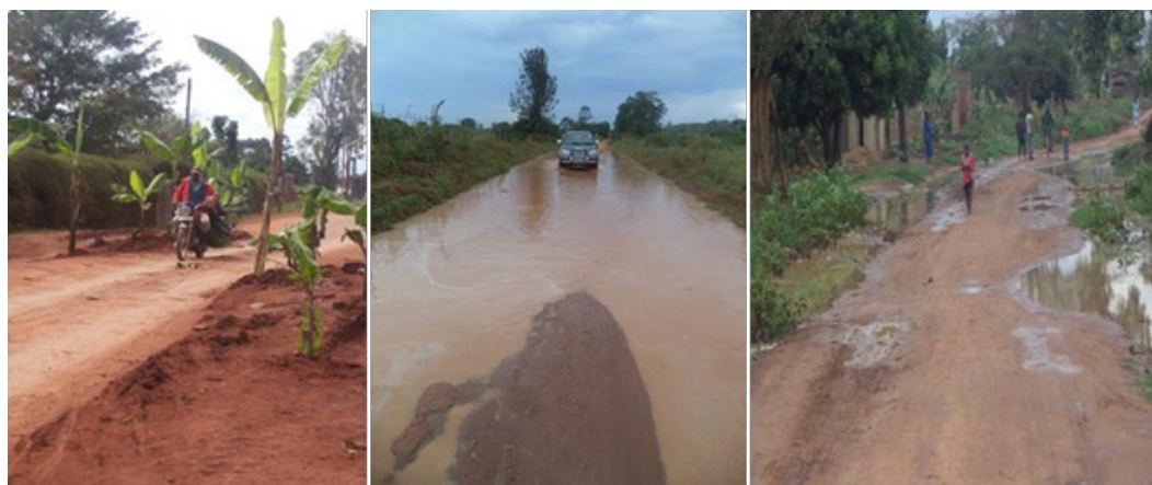
Figure 5: Poorly maintained Roads. Right: Kayabwe – Bukasa Road. Centre and Left: Sections of Kituntu – Kayabwe Road
