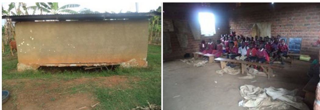
Figure 3: A Collapsing Toilet and an Incomplete Classroom Block at St Kizito-Ggolo Primary School, Ggolo, Nkozi Sub-county
