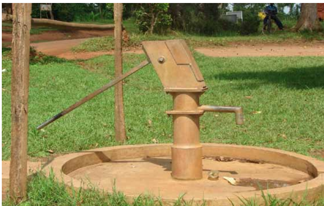
Figure 7: Non-functional borehole at Katoogo HC III, Nama Sub-county
