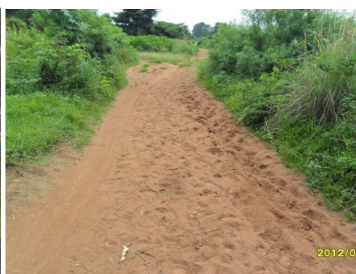
Figure 8: Road under routine maintenance
