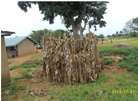
Figure 3: Improvised urinal shed at Senda Primary School
