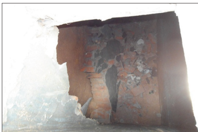
Figure 3: Collapsed inner wall of the pit latrine Pit latrine at Kihungya Primary School
