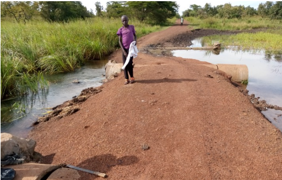
Figure 27: Broken culverts on Awuc Stream
