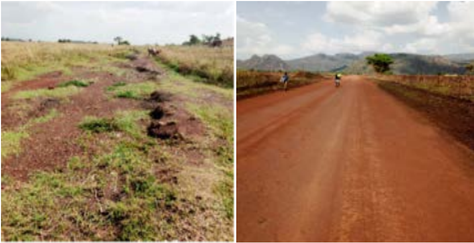
Figure 29: A section of Lomorimor road before and after Rehabilitation by UNRA
