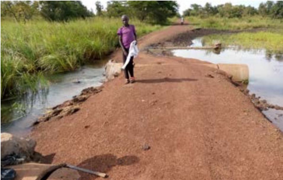
Figure 27: Broken culverts on Awuc Stream
