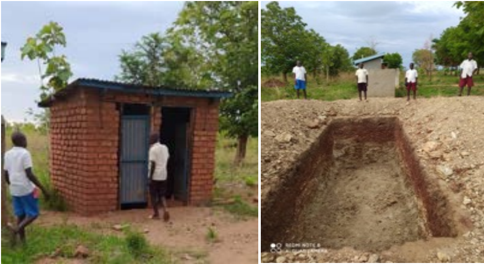
Figure 9: The only 2 Stances of boys' Pit latrine that existed in the school (L) and Pupils appreciate the process of digging the new pit latrine (R)
