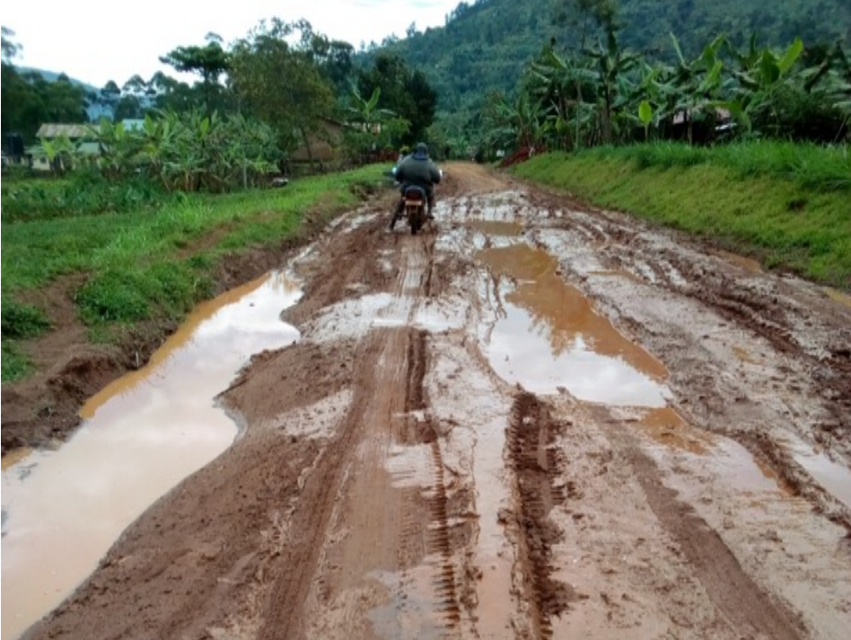
Figure 33: Bumasata – Bushiyi road at a time of conducting the CEAP meeting in Bushiyi Sub-county (November 2019)
