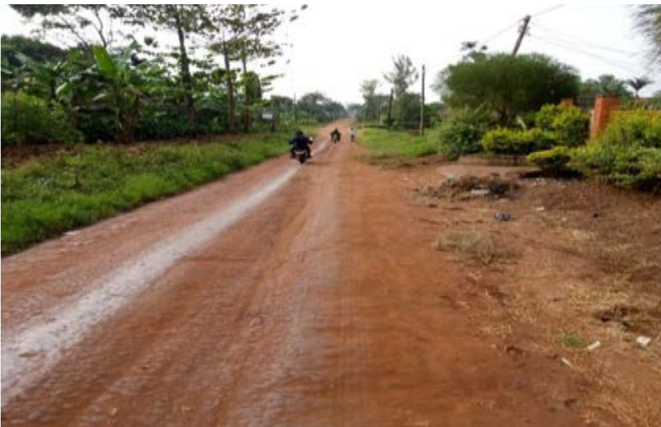
Figure 34: A section of Bumasata – Bushiyi road after repair (March 2021)
