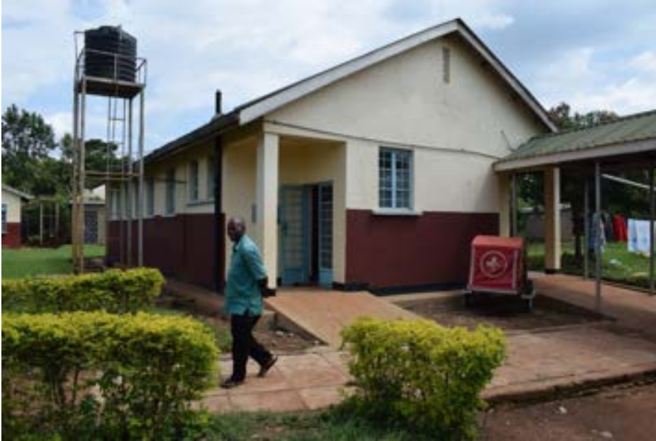
Figure 16: Photo of a Health Unit Staff walking past the renovated theatre at Nankandhulo Health Center IV taken in March 2021
