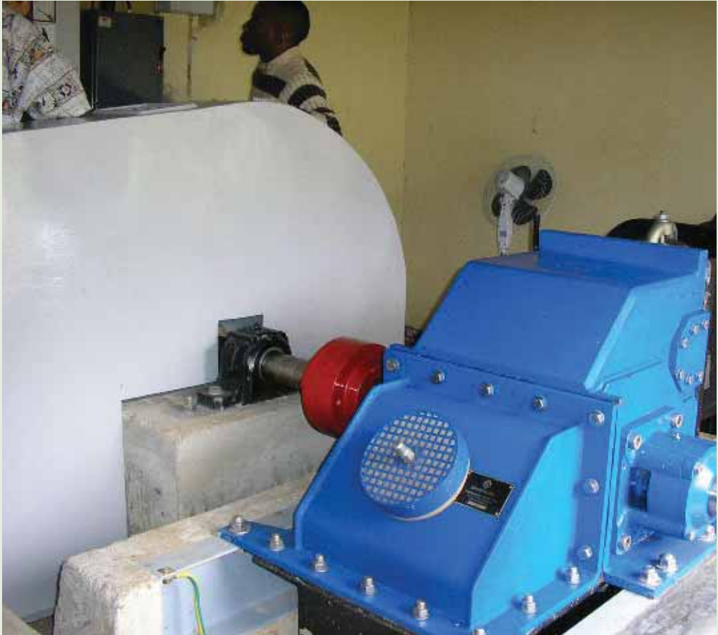
Fig 1.1: Powering the rural areas: A 55kw Pico Turbine lighting up Bwindi in south-west Uganda. (Sourec: Ministry of Energy-Uganda)
