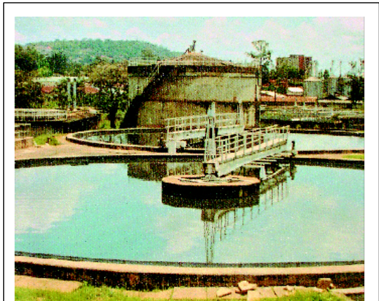
NWSC Water Purification Plant in Bugolobi: Many Agencies do not actively disseminate Information to Citizens
