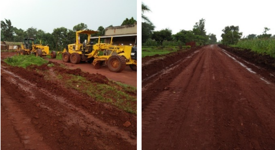
Figure 25: Grading underway on Doko to Kolony road in response to the citizen petition
