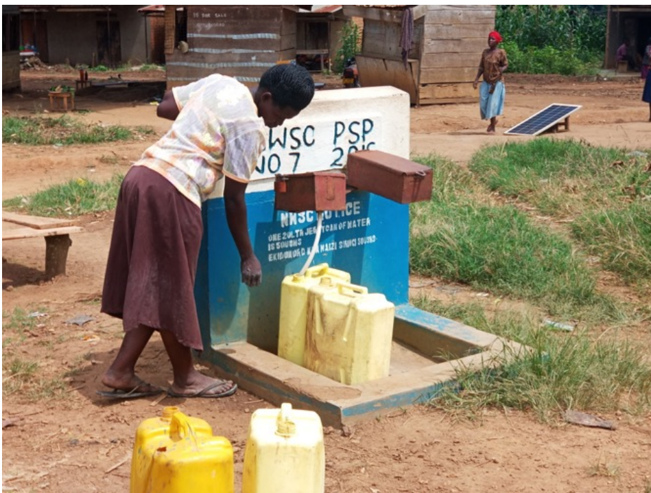
Figure 15: A resident member of Kigaju cell draws water from a newly built public water post in Kisiita Ward, Karujubu Division
