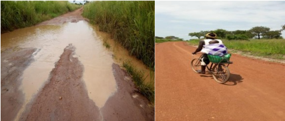
Figure 21: Goro-Poli to St. Thomas Moore road before and after rehabilitation
