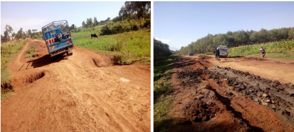
Figure 23: Bad sections of Doko to Kolony road, the basis on which citizens petitioned the district council for action
