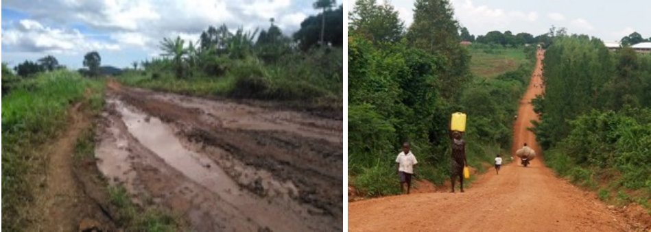
Figure 17: The bad section of Katagurukwa - Kinumi road in 2016 (L) and (R) a section of the same road after rehabilitation in June 2019
