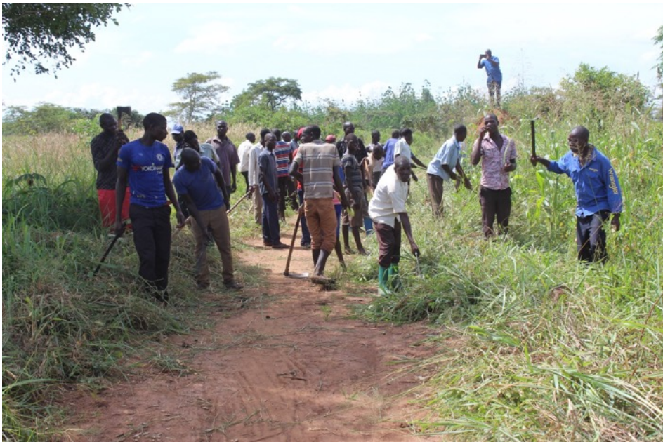
Figure 32: The youth of Abongokongo village Clearing the road linking Abongokongo to Ayumi parish
