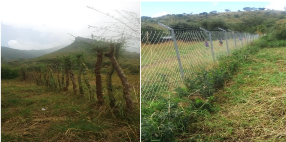
Figure 10 : Part of the school fence made of local poles & barbed wire (above) and (below) is the chain link fence on another part of the school
