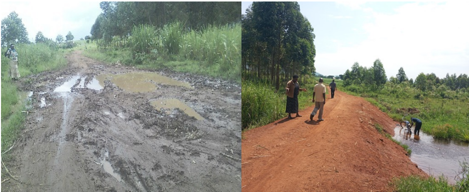
Figure 18: A bad Section of the road at Nsambya swamp in 2018 (L) and the same section of the road after completion of works in June 2019 (R)
