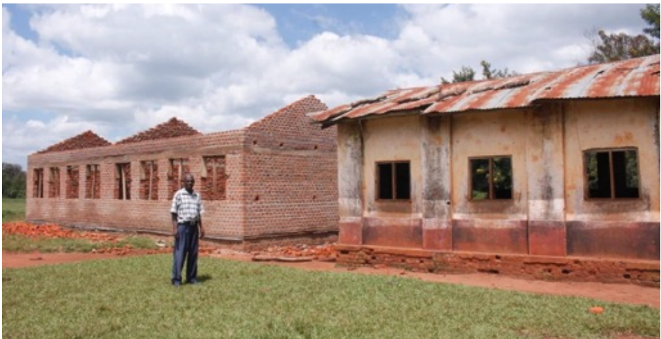
Figure 4: A picture taken at the time construction of a new classroom block was ongoing at Bugeywa primary school
