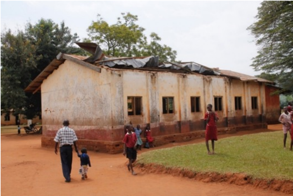
Figure 1: The roof of a classroom block blown off by strong winds
