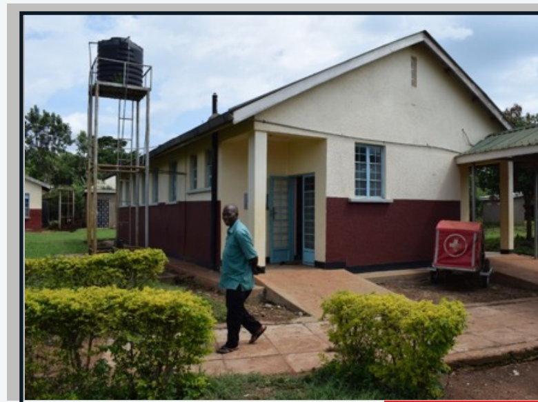
Nankandhulo HC IV After renovation
